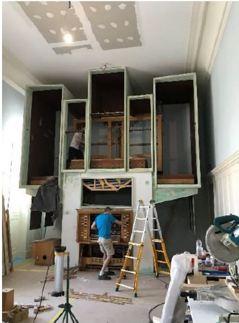
Installation orgue, salle Montillet
