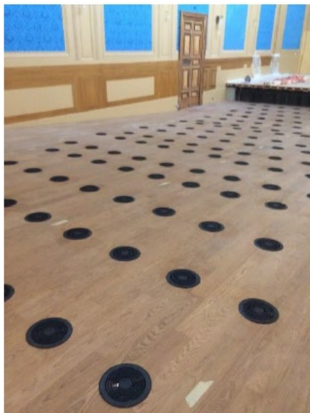
Pose grille sol grande salle
