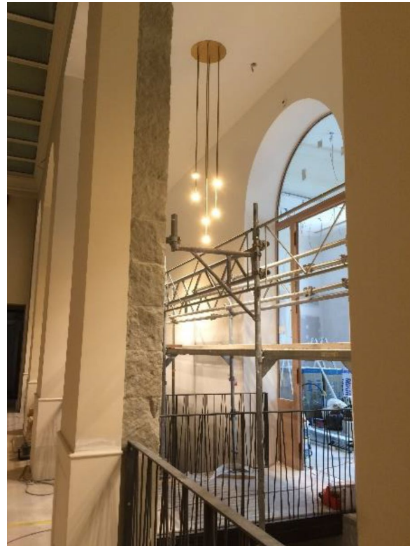
Pose luminaire atriums Calame
